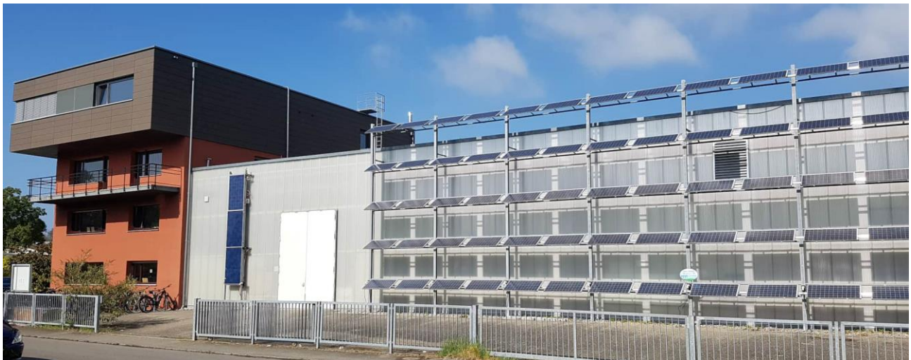
Figure 4-19: PV balustrade on ISC building (source: ISC Konstanz)
